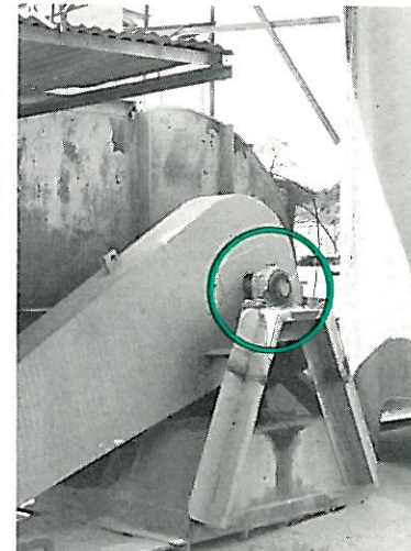
Fig. 3-3: Foote-Jones Heavy Duty Pillow Block supporting a V-Belt Drive.
